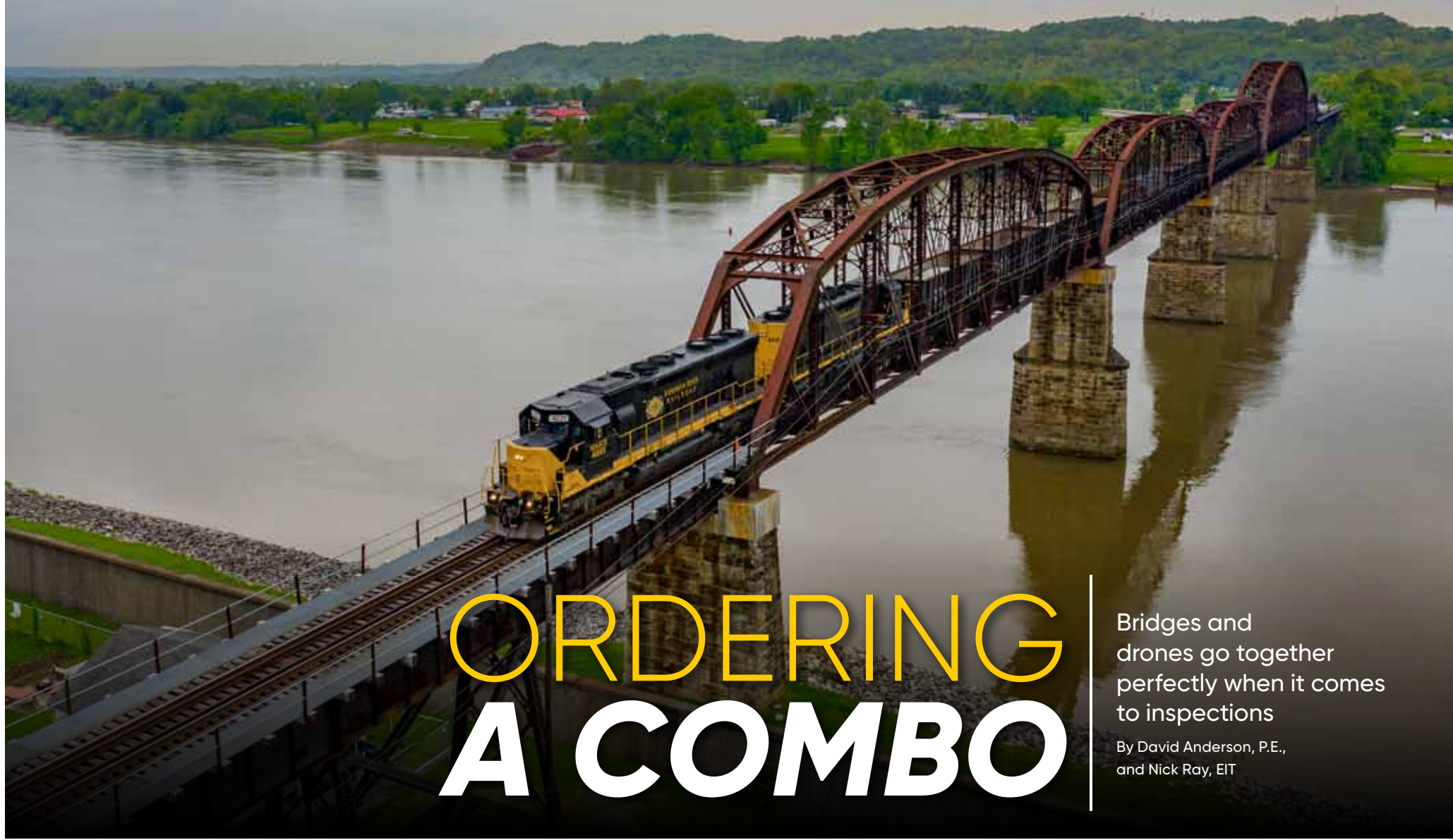
ARE used a drone to inspect the Ohio River Bridge.
